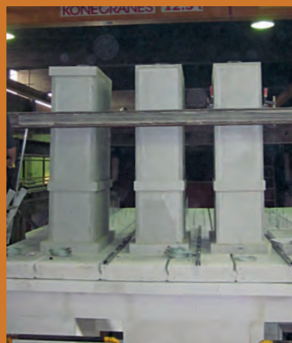
Installed service shafts
