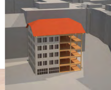
Fig. 4 (a): Example of a multi-storey wooden building with skeleton structure
