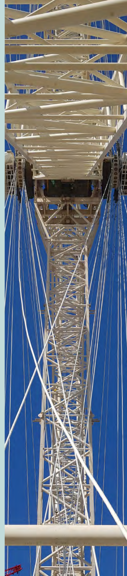
Project: Halogaland Bru, Norway Stay Cable: Fatzer, Switzerland Photo: Fatzer
