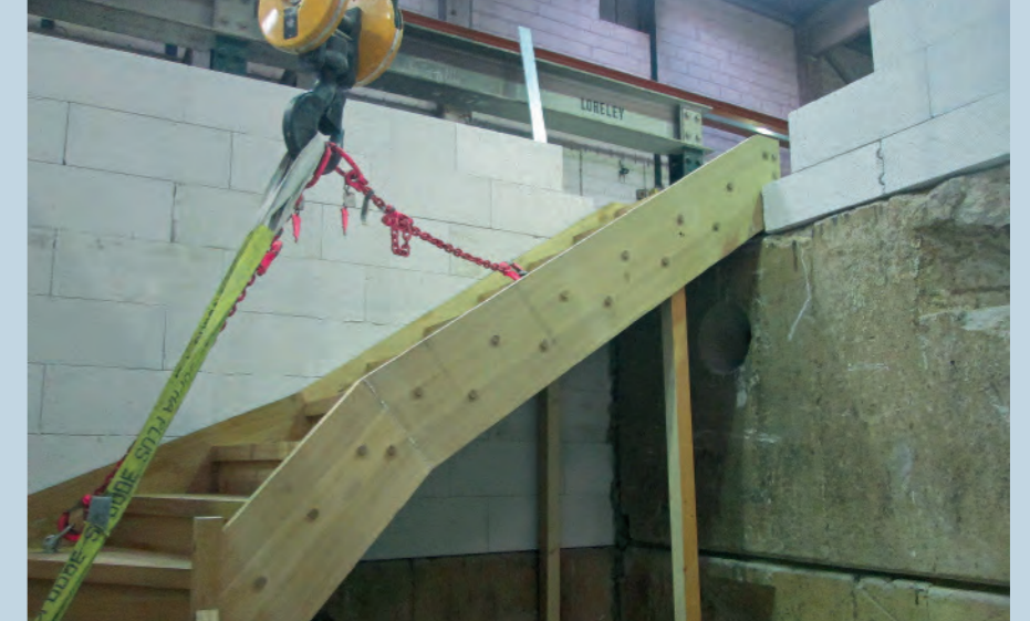
Installing the life-size, wooden staircase in the test furnace
