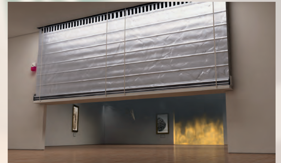
◀ Compartment-creating operable fabric curtain that wraps around a corner (photos by Stöbich Brandschutz)
