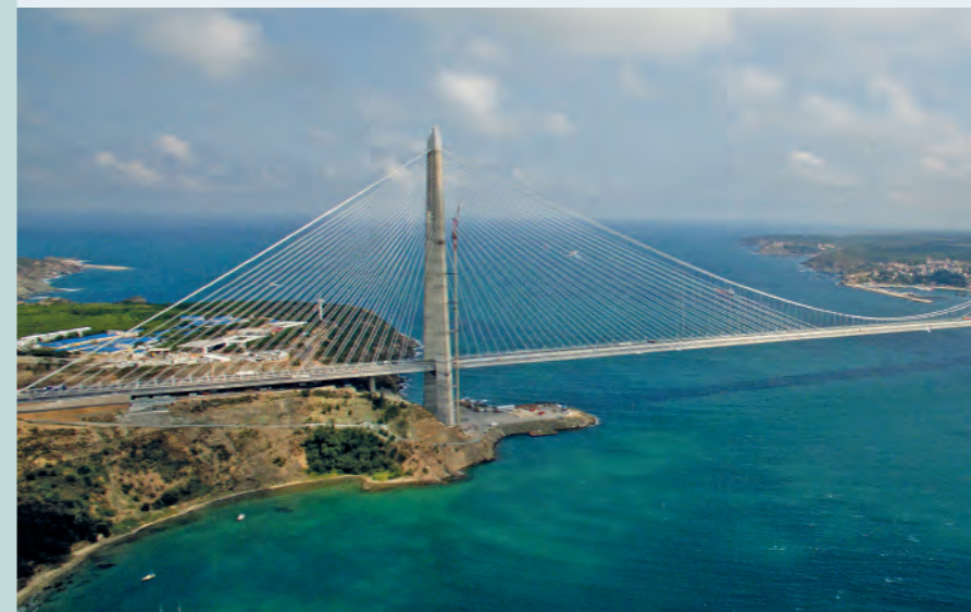
Project: Yavuz-Sultan-Selim Bridge (3. Bosphorus Bridge), Turkey Stay Cable: Freyssinet, France; Photo: Freyssinet
