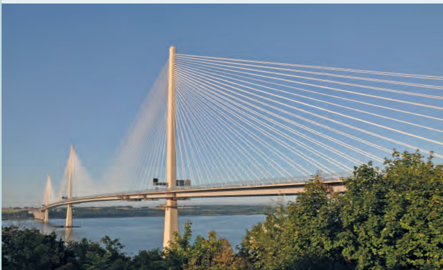
Project: Queensferry Crossing, Edinburgh, Scotland Stay Cable: VSL, Switzerland; Photo: Dr. Martin Laube
