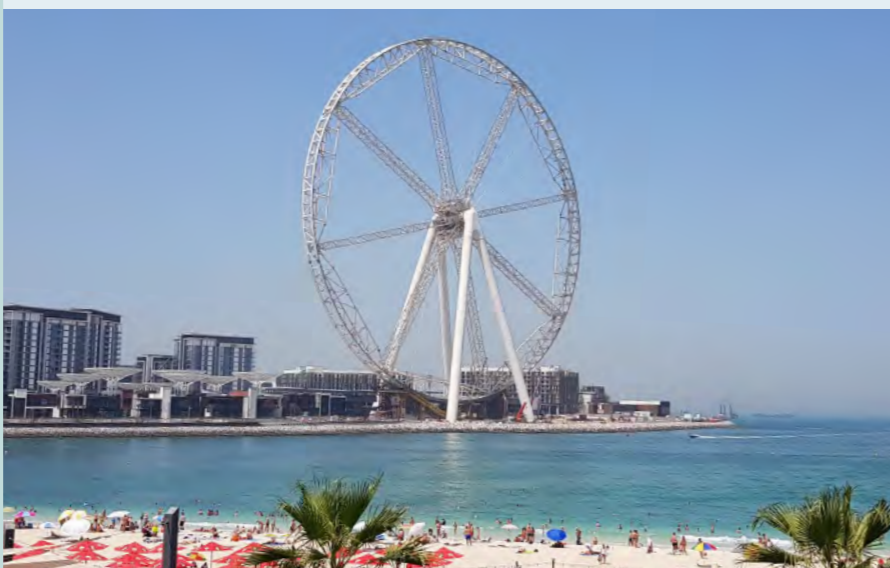
Project: Ain-Dubai, VAE Cable: Julisling, China; Photo: Beom Soo Park; Photo: Beom Soo Park
