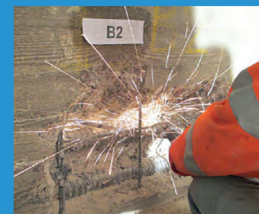
Taking prestressing steel samples
