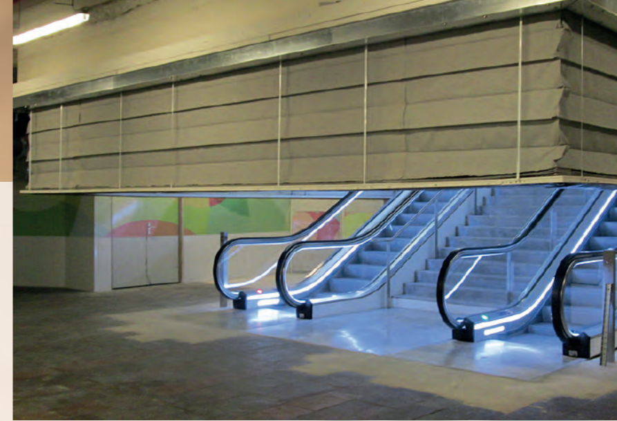
◀ Compartment-creating operable fabric curtain that wraps around a corner (photos by Stöbich Brandschutz)
